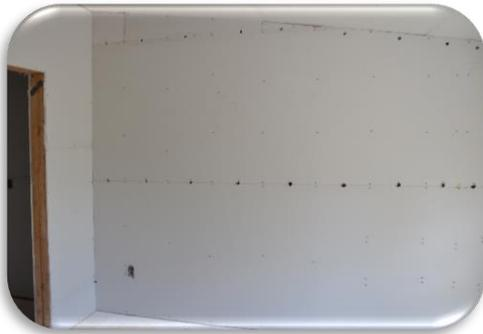
On an 8-foot wall, we recommend placing one hole at 4-foot high level on drywall seam and one hole near top section of drywall near double upper plate.
