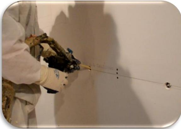
When spraying 2x4 wall cavities, you should be injecting using an AR4242 (01) Mixing Chamber and pressures between 1,000 and 1,200 psi to obtain a good mix at the bottom of the wall cavity. Make sure that the length of your tubing (4" to 6") allows you to be able to direct the injected foam towards the bottom of the stud cavity.
