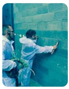
Clean the fill holes with a drill/wire brush attachment to insure a clean hole before patching. The GacoProFill foam is very easy to clean and remove from concrete block.
