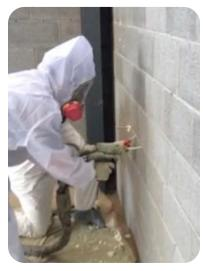
With pour cap and tube installed on gun, place tube into cavity working from the bottom of the wall up, taking care to fill each and every cavity. Again, a check with a thermal camera helps ensure every core cavity is being filled. A record of the thermal images can also be recorded for the building owner as a proof of performance for the project.
