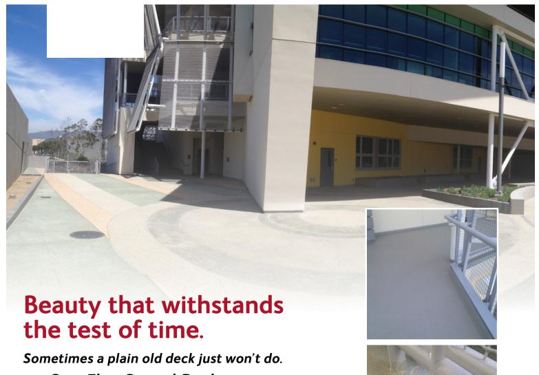
With **GacoFlex Crystal Deck**, you can create a customized look for your deck that makes you stand out from the crowd. Crystal Deck is a seamless membrane pedestrian deck system that incorporates colored crystal quartz granules for added slip resistance and a customized look. With a variety of available color combinations, Crystal Deck is the most versatile of Gaco's decking and waterproofing systems – limited only by imagination.
